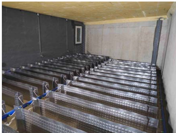
Figure 8: Left: Part of the section of the building. Highlighted are the ice storage next to the underground car park and the collector field on the flat roof. Right: Photo of the ice storage with 210 m 3 volume before filling. At the bottom heat exchangers are installed that can be de-iced.
