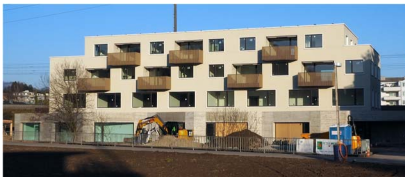
Figure 7: New building with 2'050 m 2 of floor area which is supplied with heat by the solar-ice system.
