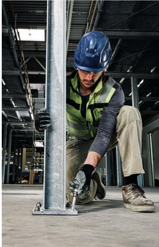
Columns and beams
