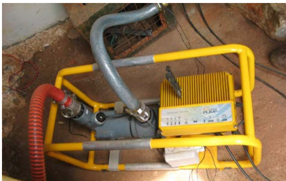
Figure 20: Ennos Sunlight pump installation
