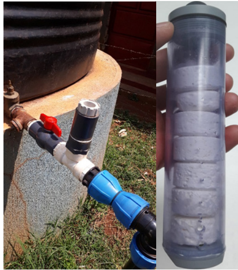
Figure 67: T-chlorinator and cylinder
