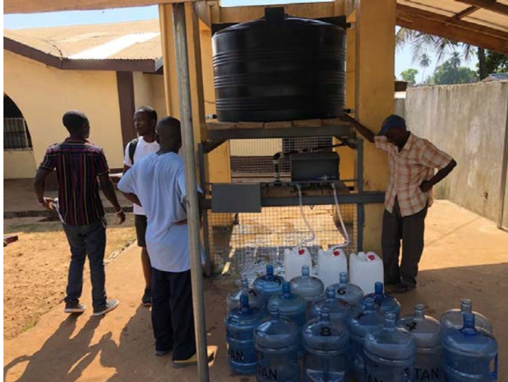
Figure 46: Water taps at the vertical GDM system in Liberia
