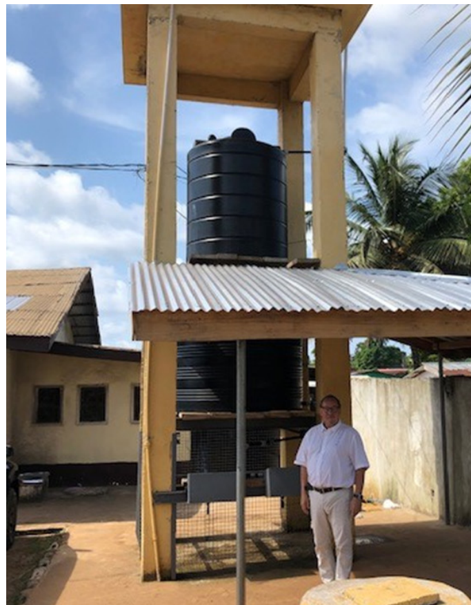
Figure 40: Picture of vertical GDM treatment system
