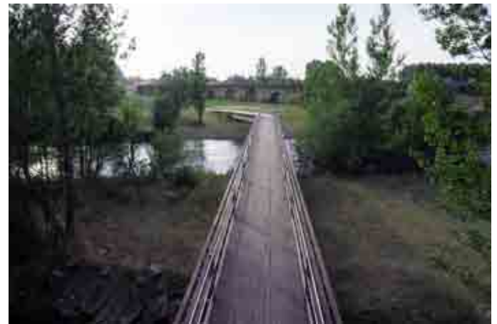
FIGURE 4. Image of the footbridge at Puente Villarente, Spain. (LABPAP, 2010)
