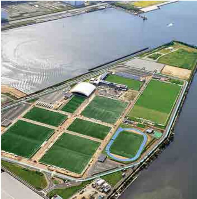
FIGURE 4. The site is now redeveloped into training centre for football 4 (Author: Showa Sekkei)
