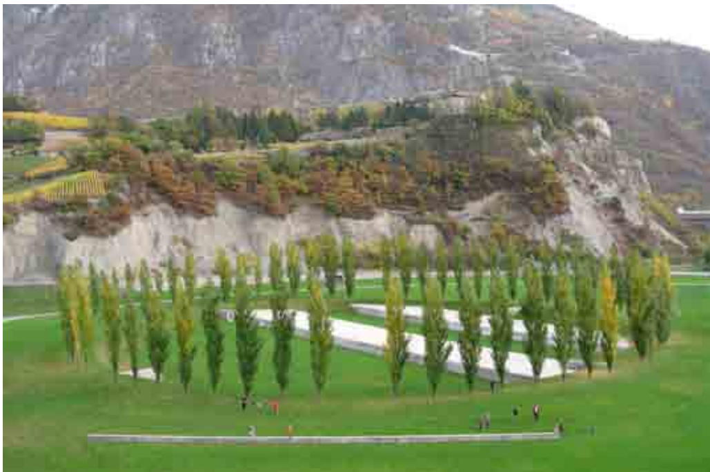
FIGURE 2. ESPACE AUGUST PICCARD photo Studio Bürgi The crossing of a new motorway in this landscape offered the chance to redesign a place, to rediscover it with the language of the essential. The two enclosed tunnels 'reappear' in a sculptural space, a place for meetings and confrontations with our time, recreation, exhibitions, festivals or just a place to reflect, or for a moment of desired solitude.
