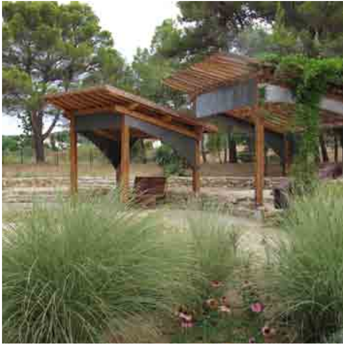
FIGURE 1. Shade structures at the Rab Psychiatric Hospital. The stone walls are an important cultural symbol on the Adriatic islands and were requested by the community.
