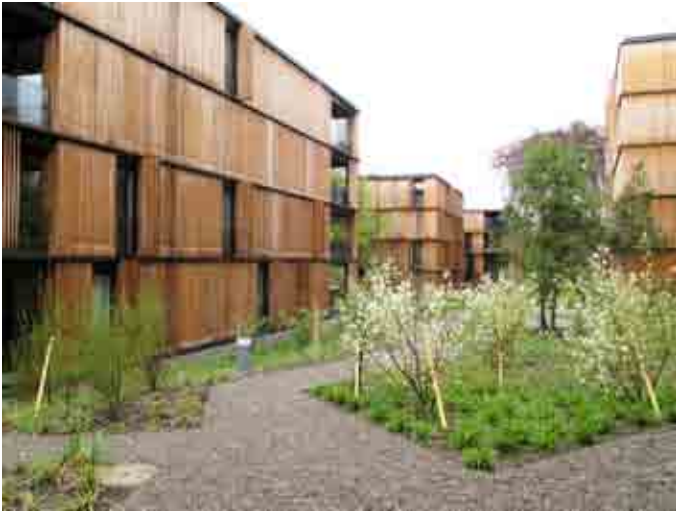
FIGURE 1. Residential environment designed according to ecological criteria with integrated mature tree population. Siedlung Escher Park in Zurich. (Photo U. Liemdb)
