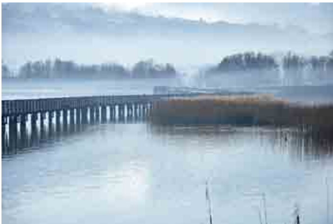
FIGURE 2. View of Rapperswil-Hurden footbridge, Switzerland. (Roland zh, Wikimedia Commons 2011)
