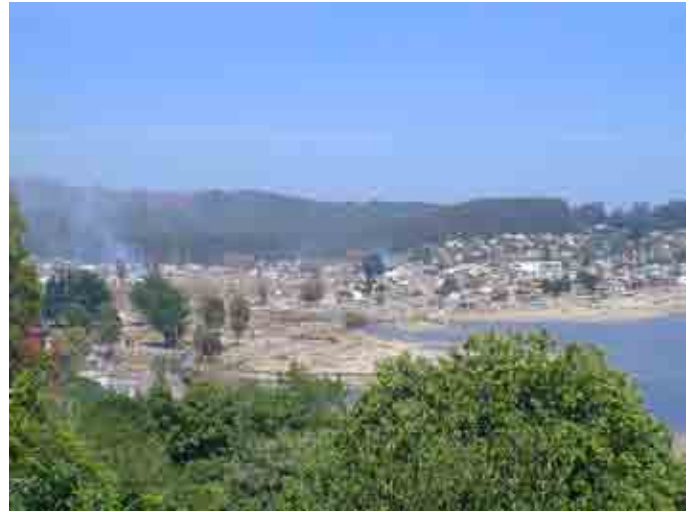
FIGURE 2. Dichato, VIII region, Chile. 2010, a few days after tsunami. Courtesy of Mario Torres Jofré, Architect.
