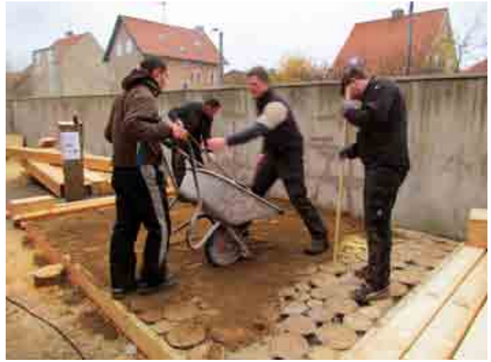
FIGURE 2. Wood is being assembled into terrace floors.
