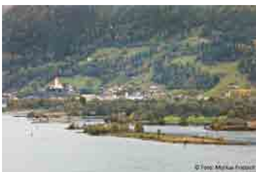
FIGURE 5. Islands in the Reuss delta (UR) constructed of excavation material from the Gotthard tunnel. Some of them protect the fragile bank, others give space to bathers or nesting birds and creates multifaceted habitats (design: Team Landschaftsprojekt Reussdelta). © Markus Frietsch
