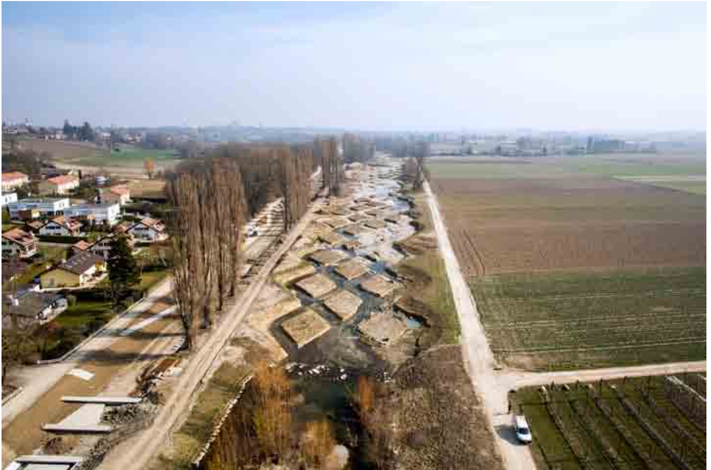
FIGURE 3. SUPERPOSITIONS, (Georges Descombes, ADR et al.), L'Aire, Geneva, Switzerland, 2001–2016. Earthen lozenges were excavated from the river bed, to erode over time as vegetation takes hold. (Courtesy SUPERPOSITIONS, 16 March 2015)
