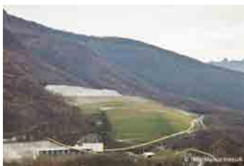
FIGURE 4. An artificial mountain in the forested hills, mounted up of 3.5 million cubic meter rock excavation in Sigrino (TI). In accordance with the solid tradition of Swiss design there was no attempt to present something artificial as natural. The landscape design developed its forms and material use from the dialectic between the natural and artificial (design: Atelier Girot). © Markus Frietsch
